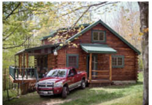
Roof and Trim: Evergreen
