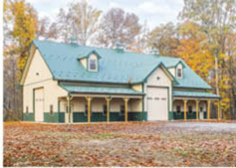
Roof: Evergreen Sides: Light Stone Trim and Wainscoting: Evergreen
