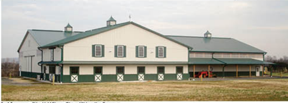
Roof: Evergreen Sides: Light Stone Trim and Wainscoting: Evergreen
