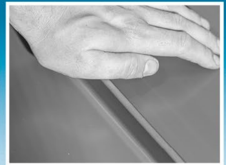
Snap the next panel in place.
