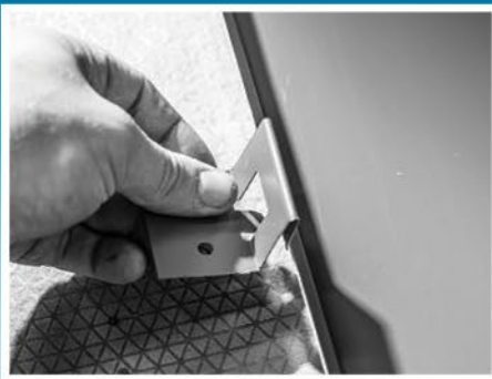
Attach the hidden clip to panel.
